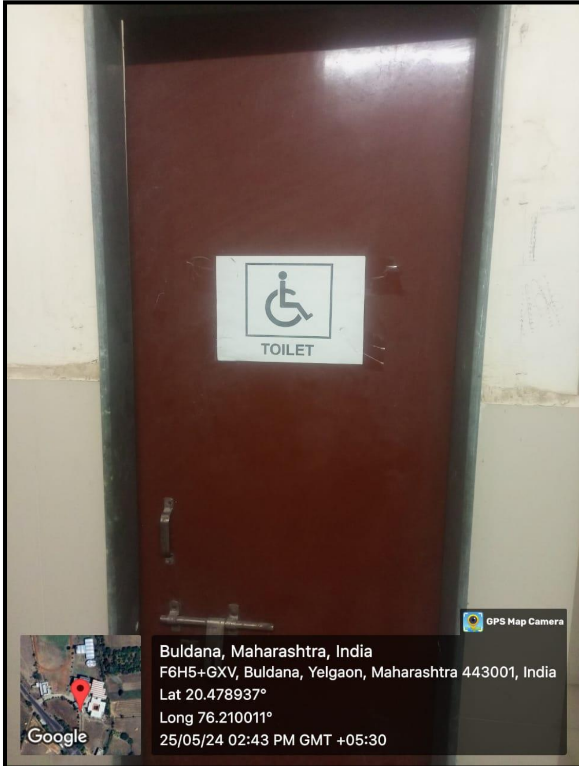
Separate arrangement of toilet for Disable Person
