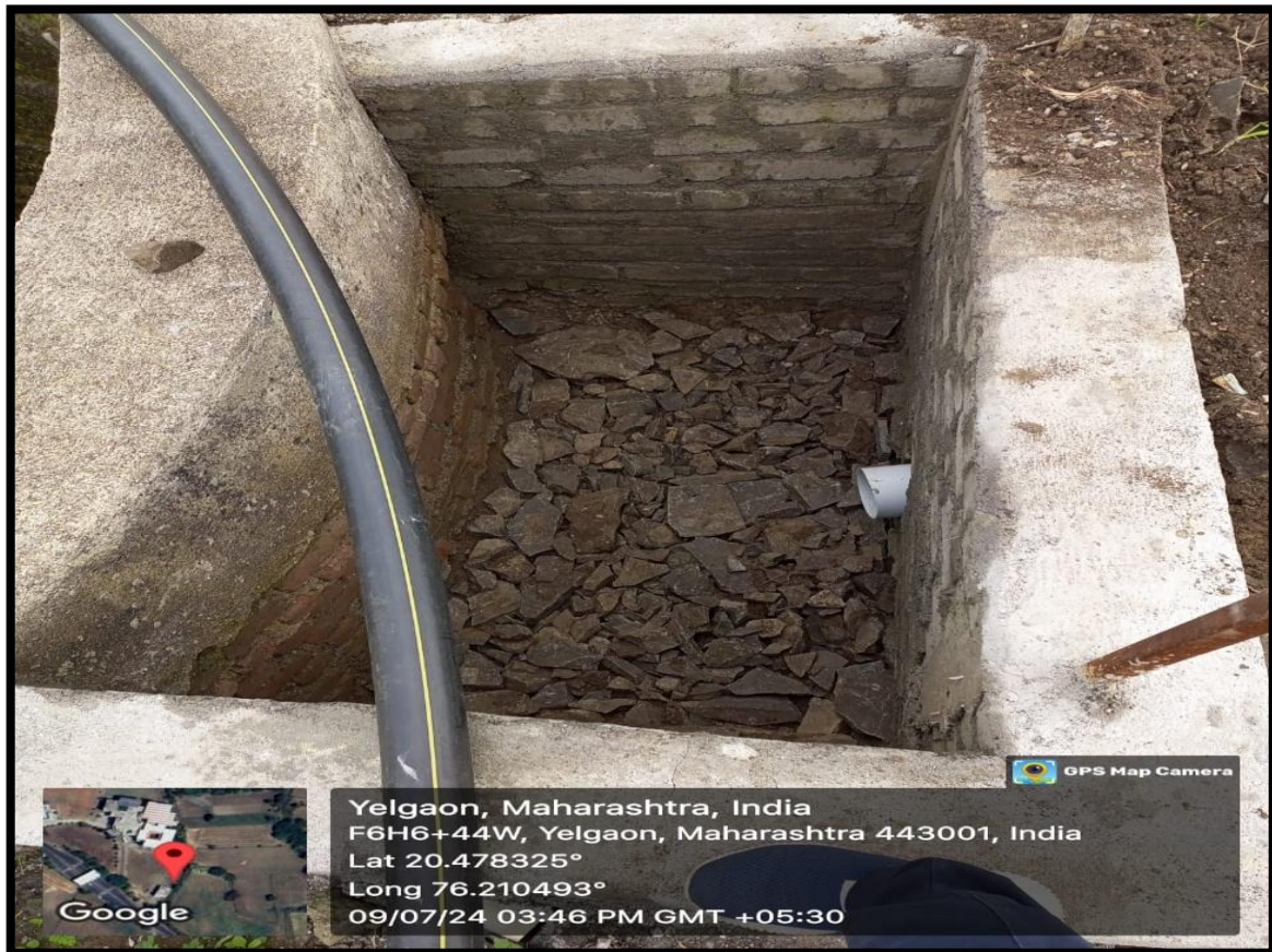
Rain Water Harvesting Pit
