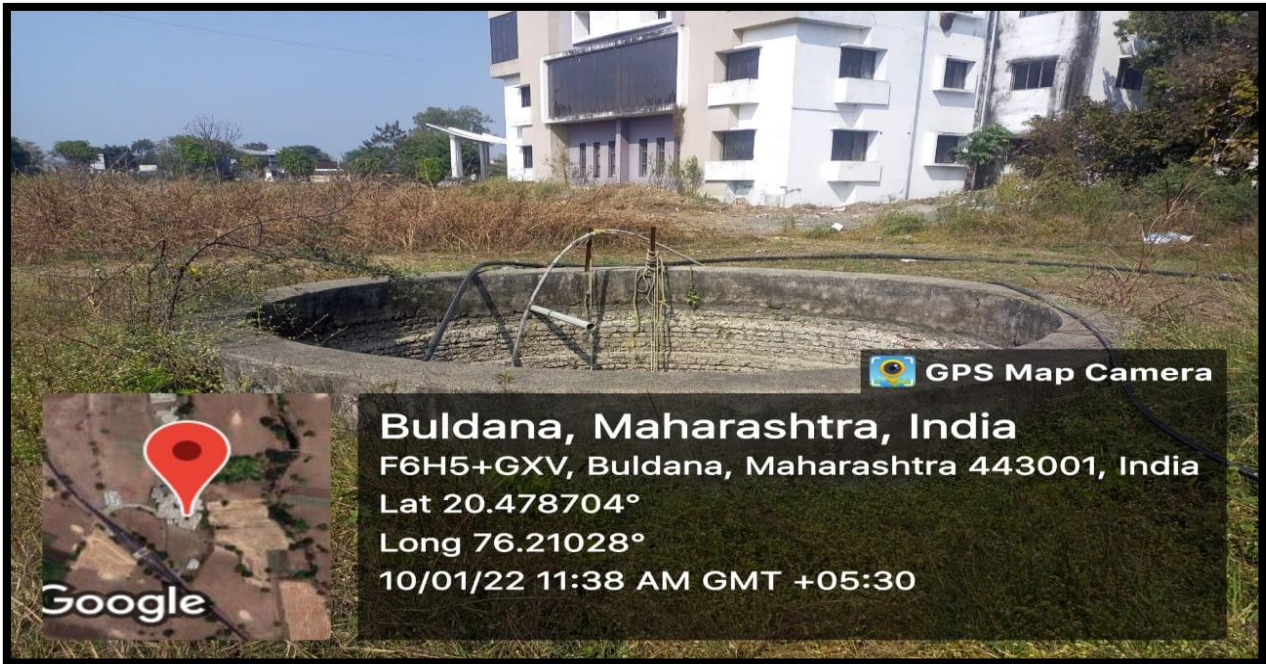
Two Water wells available in campus
